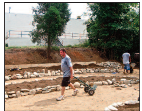
September: Slow Food volunteers and contractors transform the space.
